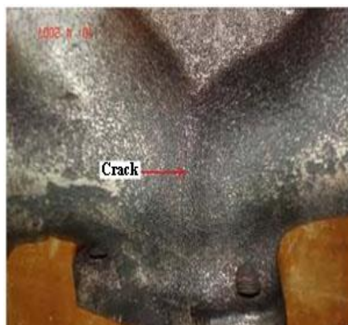
Figure 10 Hair-line crack in thermal shock test [35]
